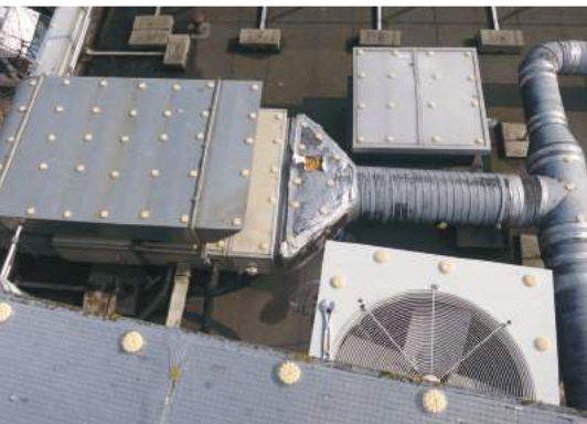
Evenly-spaced dishes protect HVAC equipment on a building roof.
