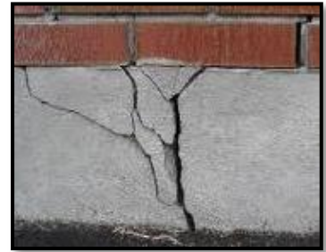
Foundation Cracks
