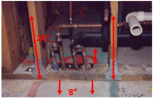
Typical bath trap areas for treatment: Treat sill plate, up studs 24 inches and 8 inches out onto slab from the sill plate
