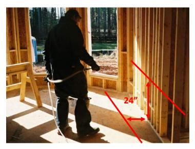
Treat framing and the flooring upon which it is attached in a continuous 24 inch band
