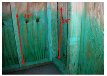
Treat from the sill plate up 24 inches high and 8 inches down on the block or slab. Typical treatment is between the red lines or as indicated by the green dye to the right.
