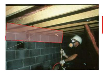
Treat eight inches down on the block and 24 inches out on the joists and subfloor
