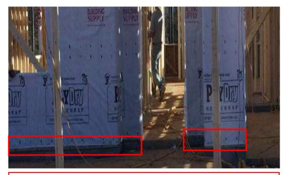
Take note of the thin strip of exposed wood between the house wrap and sheathing – be sure to treat this area so that a continuous barrier occupies any potential gaps. Lift the wrap to spray a continuous barrier up the sheathing to a height of 24 inches.
