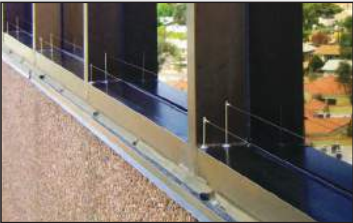
Bird Wire installed on window ledges
