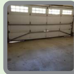
Garage Door Openings
