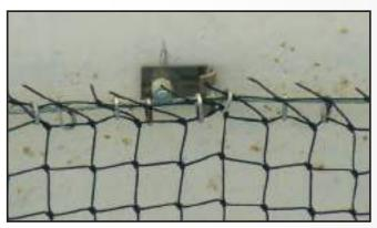
Intermediate attachments are used to secure your cable around a netting installation to prevent gaps where birds could enter. We offer intermediate attachments for wood, steel, concrete and masonry.
