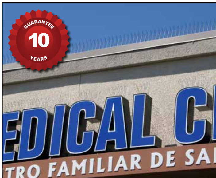
Bird Spike 2001™ installed over channel letters and parapet wall.
